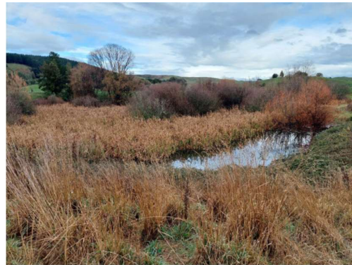
Mix of Raupo and Willows at the top end of the dam.
