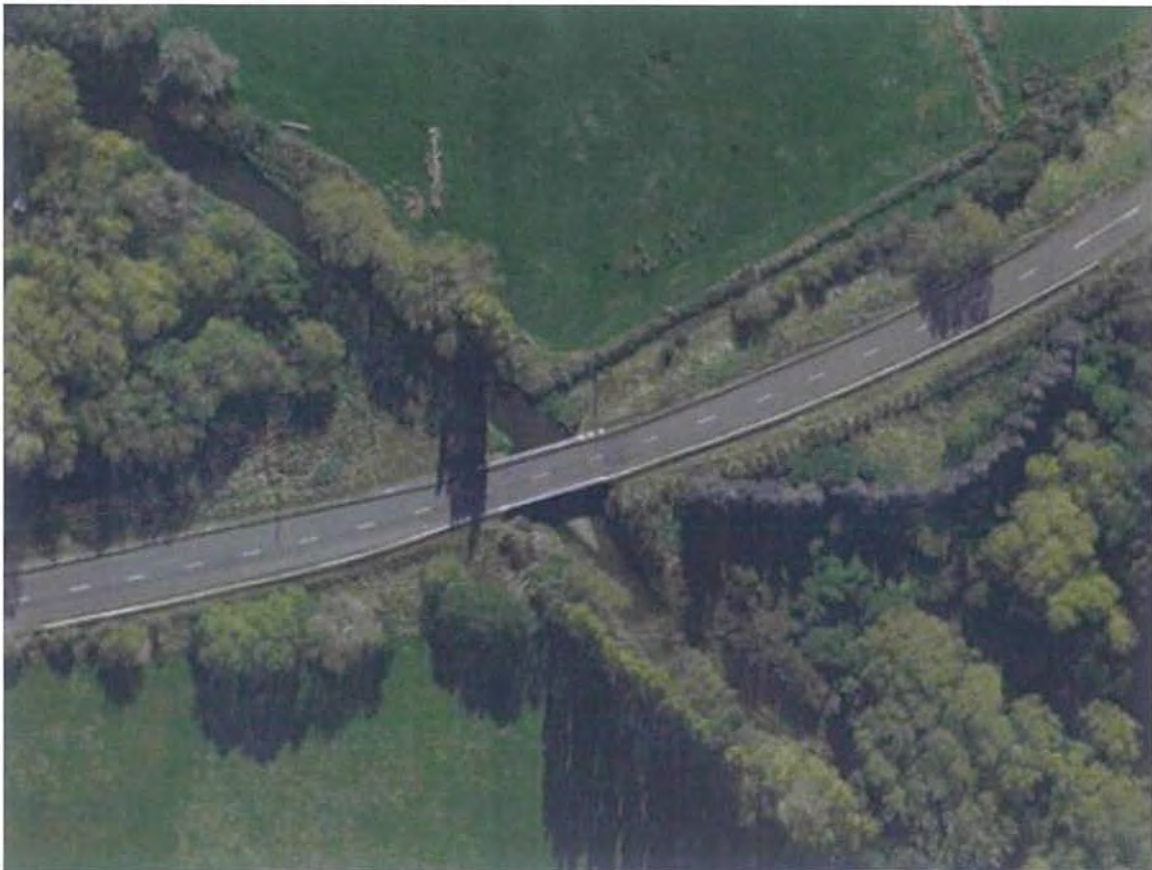
Glenure Bridge - BEFORE
