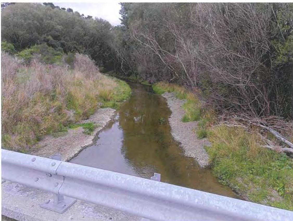
Glenure Bridge – AFTER Looking Downstream
