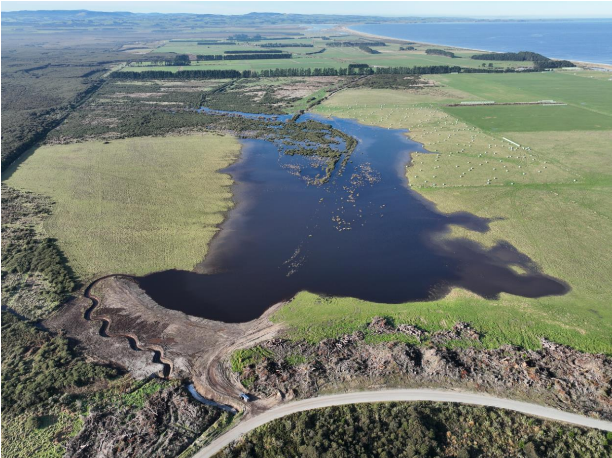
Eastern Wetland looking towards Fortrose. Note meandering outlet to provide for low gradient fish passage.
