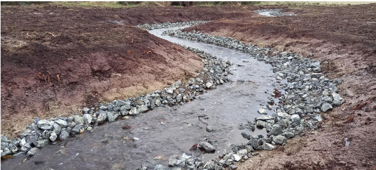
Recently-rocked meandering overflow, enabling future fish passage
