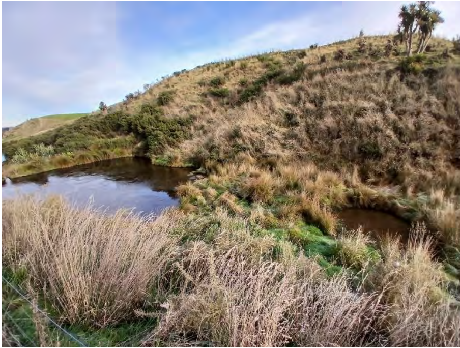
Photo 17. Shows the aftermath of wetland development, featuring two sediment traps that were constructed. The hillside in the background has been retired from grazing. The main pond is situated behind the dam wall to the left.
