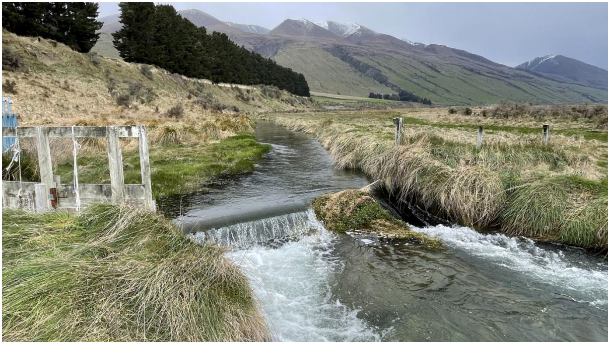
Figure A11: An intake weir on Glenariffe Stream, 80 m upstream of its confluence with Double Hill Stream.
