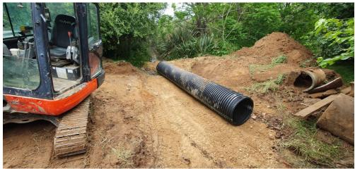
Figure 1: broken concrete culverts being replaced.
