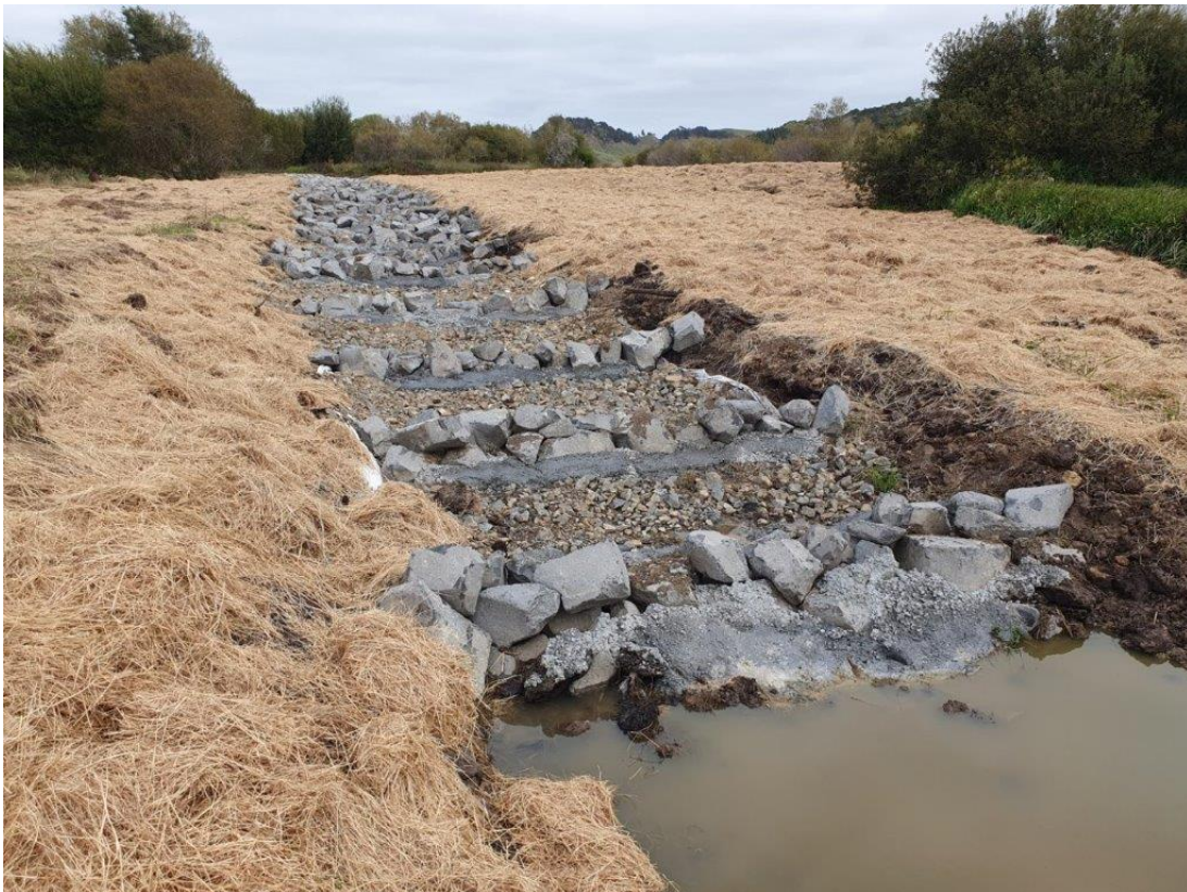
Figure 2: Fish friendly weir structure.
