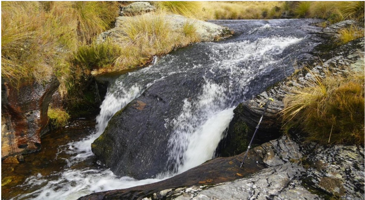
Photo 4: Hydraulic trout barrier in Armstrongs creek within the proposed footprint, around 720m altitude. Walking stick on image right for scale (I. Hadland).
