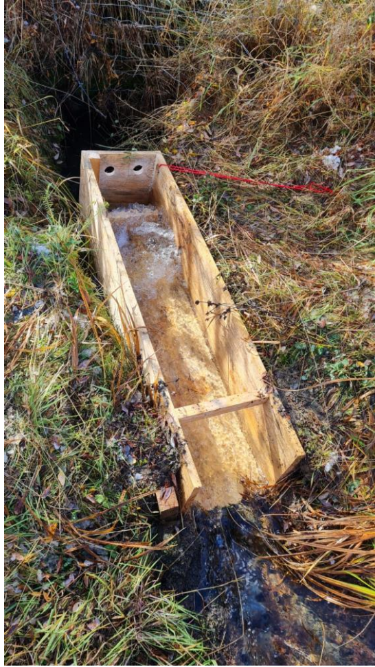
Figure 1. Temporary Fish barrier installed in Tyre Gully, Cardrona River catchment.
