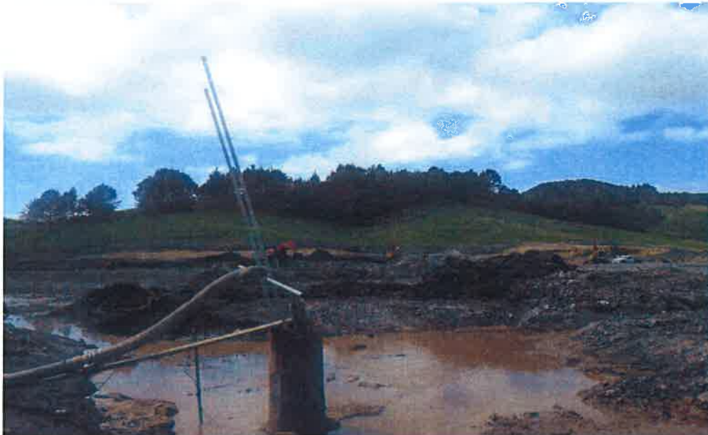
Figure 1: Earthworks commencing on the Evans Rd wetland
