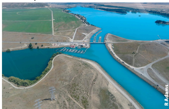
SH8 crosses the Ōhau B Canal, salmon farms can be seen on the canal and Lake Ruataniwha is in the background
